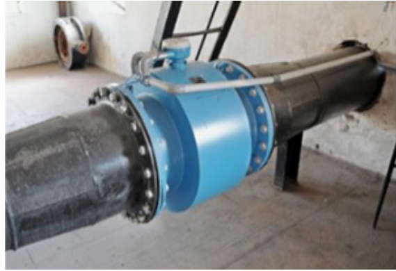
Figure 9. Magnetic flow meter (right) and sonar flow meter (left)
