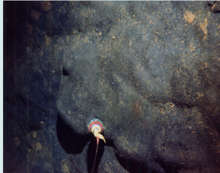
Figure 6: Crust area: covered by crust.
