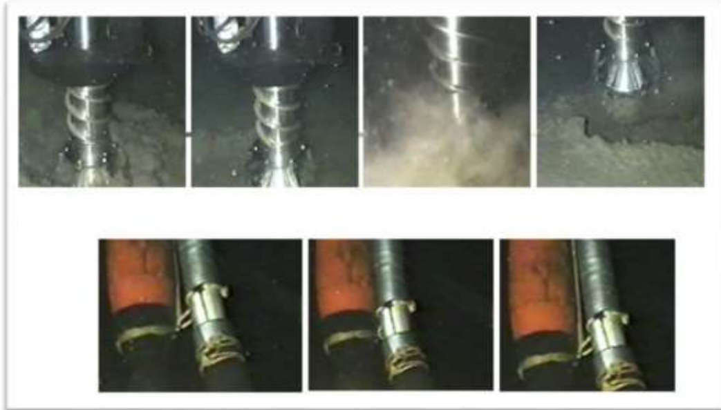
Figure 6: Initial pumping of clear water and collection of slurry
