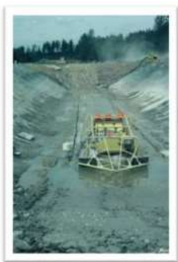
Figure 6: Electro-hydraulic collector after test run in tow facility
