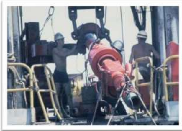
Figure 10: Dump valve being lifted to rig floor
