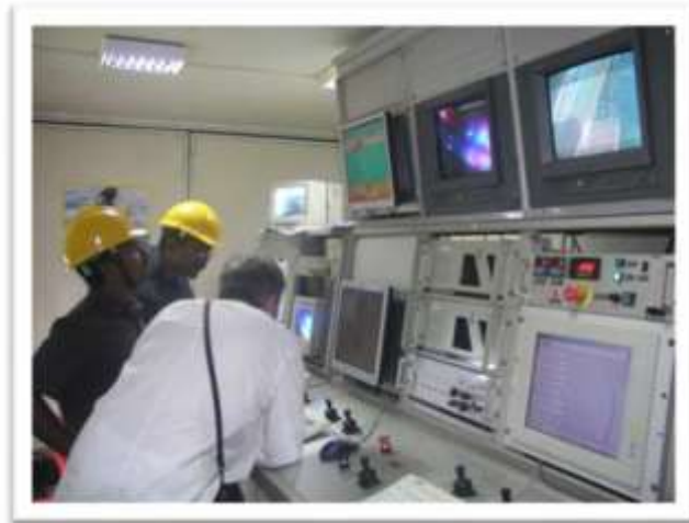
Figure 11: Control panel for in-situ soil tester
