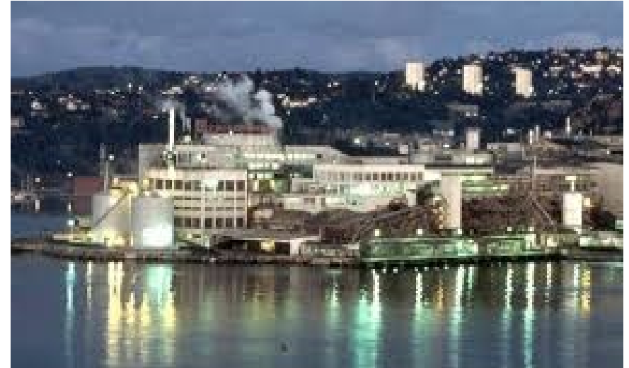
Nikkelverk Ni/Co/PGM Refinery (Norway)
