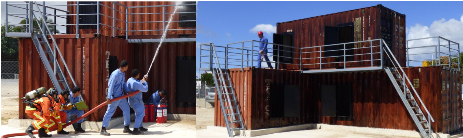
Capacity Building Programme for TMPI – TOML/NMT donated the funds (T$78k) in 2013 to build the Fire Fighting Simulator (FFS). Above photos shows the completed FFS being used by TMPI students for the first time in 2015.
